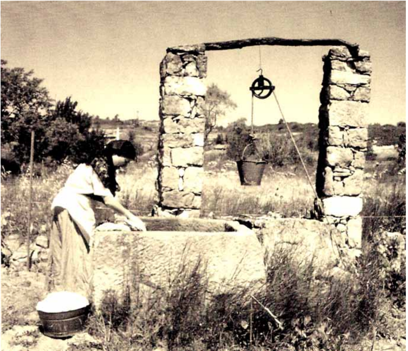
■ Water drawn from a well with a pulley was enough to fill the adjacent trough. Animals drank from them, gardens were watered, and it was even possible to do the washing, maximizing usage of water resources (Maials district limits). MUNICIPAL ARCHIVE OF TORREBESSES.
