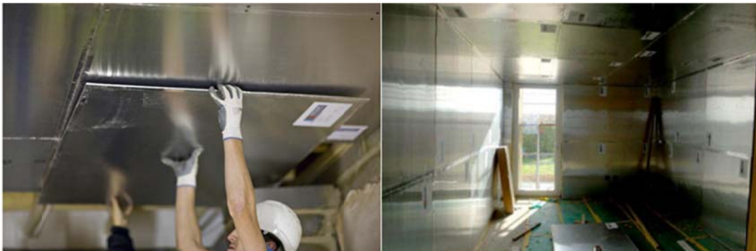
Figure 3. DuPont™ Energain® installed into the ceilings and walls [75].
