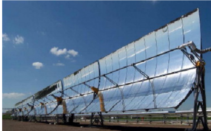
Figure 3. CSP plant from the study of Piemonte et al. [62]: solar parabolic mirrors and receiver tube (Source: [62]).
