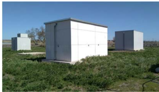
Figure 1. Cubicle used for experimentation of a radiant wall performance. Experimental test-site belonging to University of Lleida and placed in Puigverd de Lleida (Spain)
