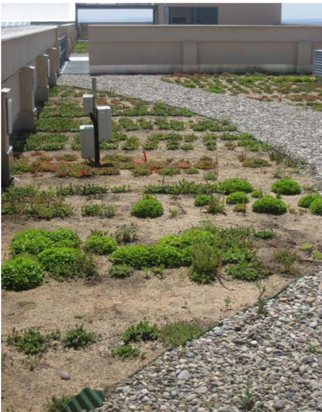
**Fig.2** Partial view of Gardeny extensive green roof. Green and gravel areas
