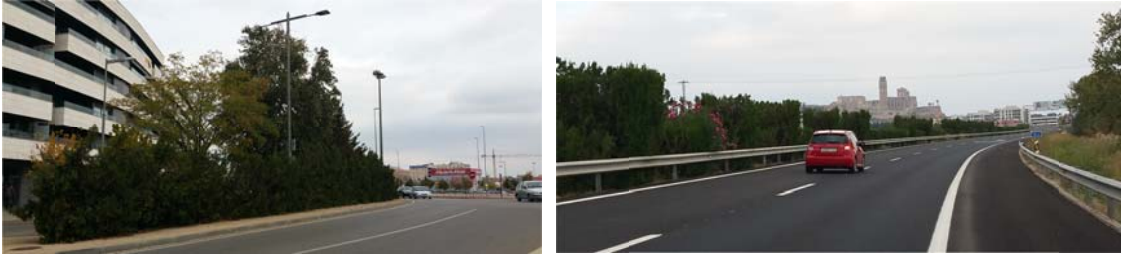
Figure 2. Road traffic noise shielding by vegetation belts
