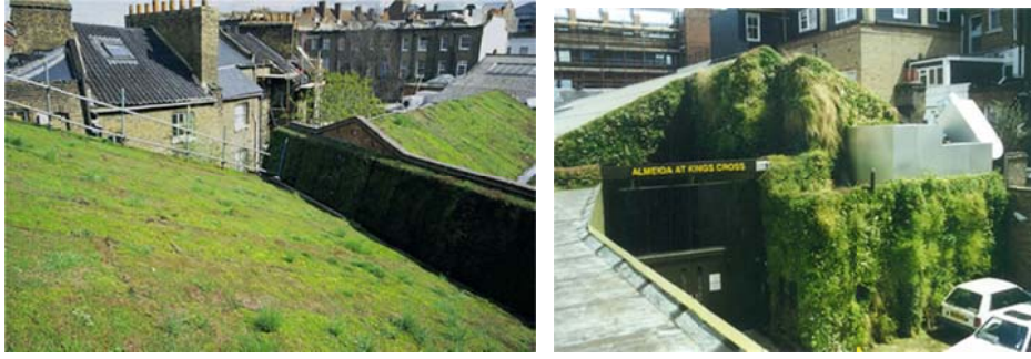
Figure 1. Building greenery as acoustic insulation. Almeida Theatre. London
