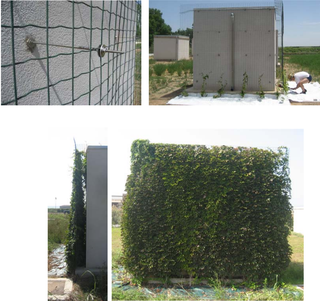
Figure 6. Double-skin Green Façade made with wire mesh and Boston Ivy
