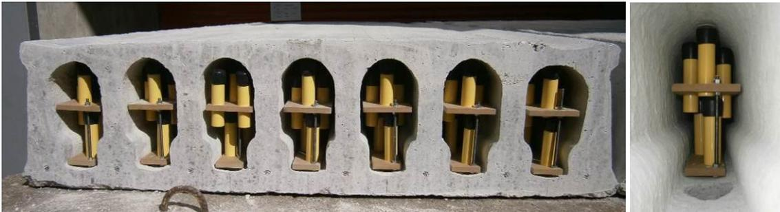
Figure 2. Prefabricated concrete slab filled with PCM tubes.
