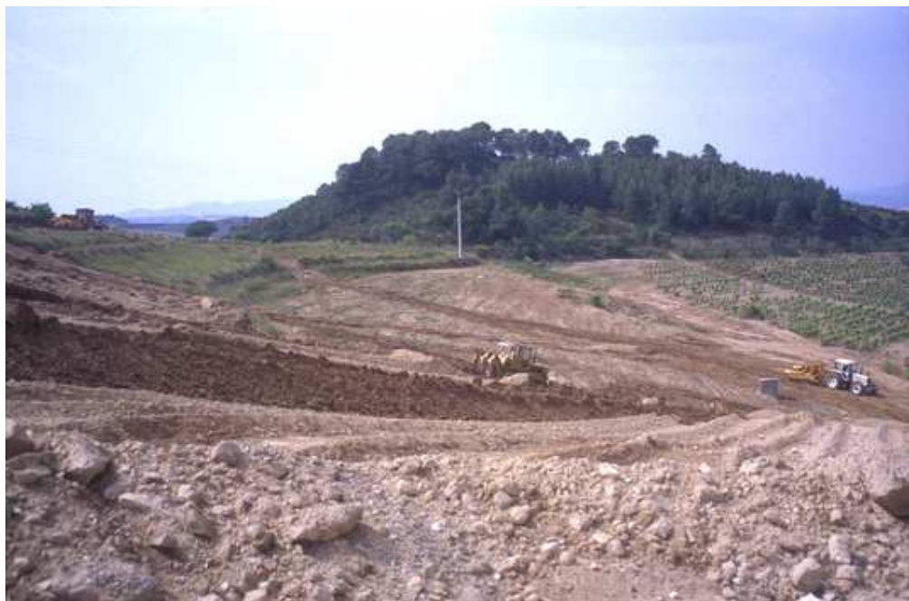
Figure 2. b) Land levelling in the Penedès region to adapt vineyard to mechanization. 22x14mm (600 x 600 DPI)
