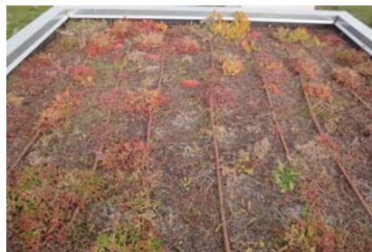
Figure 13b. Extensive green roof. Winter view (2011 to 2012)
