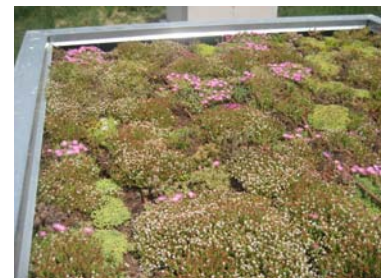
Figure 13c. Extensive green roof. Summer 2012 view. 85% plant coverage.
