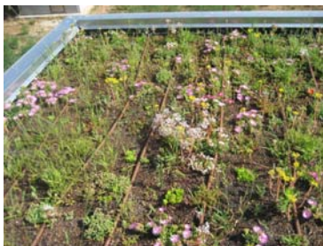
Figure 13a. Extensive green roof. Growth phase during the first summer (2011). 20% plant coverage.
