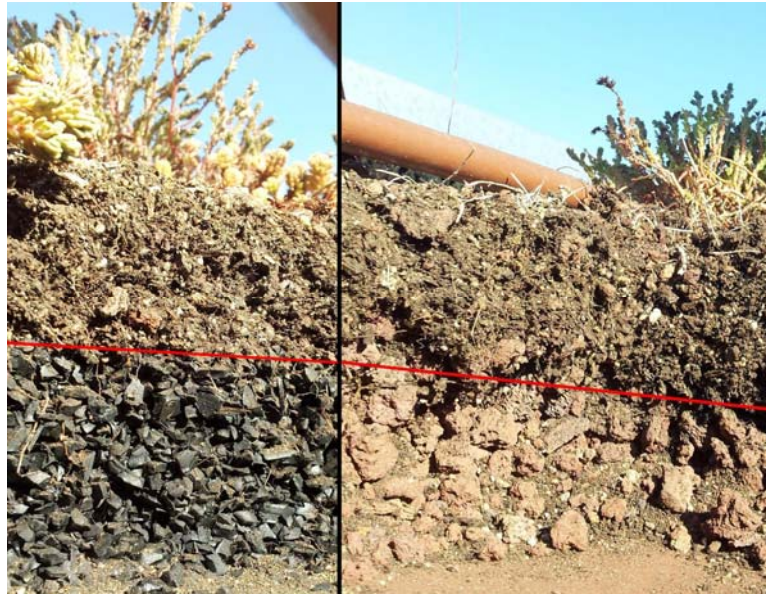
232 233 Figure 4. Stratigraphy of the substrate and drainage layers (rubber crumbs on the left and pozzolana 234 on the right) three years after their implementation 235
